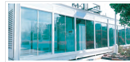
SAIC-GM-Wuling 1MWh Step-Utilization ESS Project
