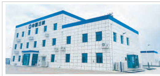
Ulanqab 180MWh Green Power Station Demonstration Project
