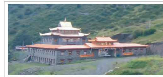
Kangding 392kWh Photovoltaic Off-grid Energy Storage Project
